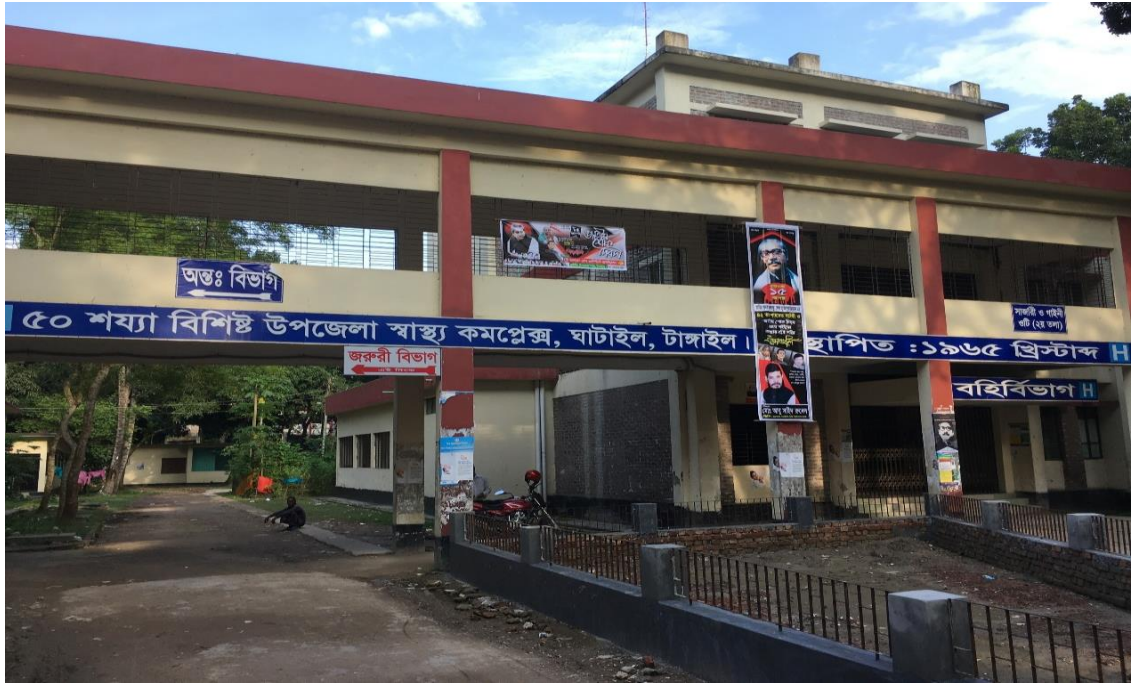
Upazila health complex, Ghatail (Source: Field data, 2017)
